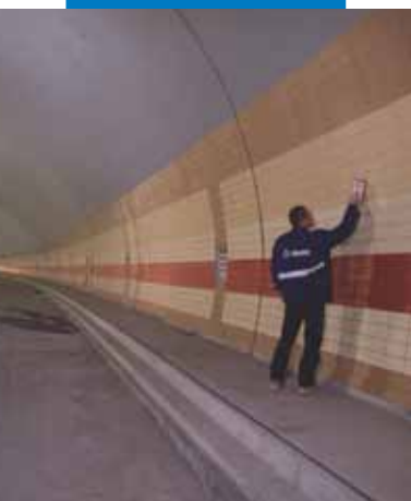
Mrázovka Tunnel - Prague - Czech Republic
