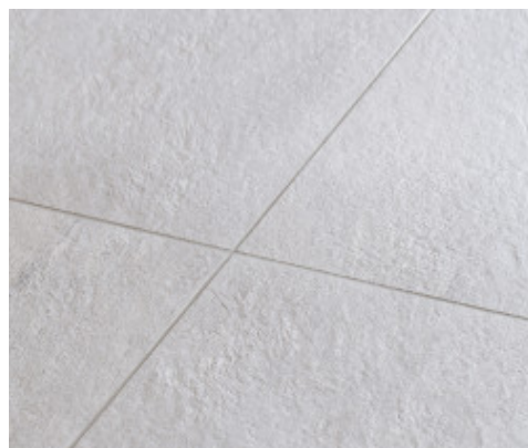
Floor grouted with Keracolor GG
