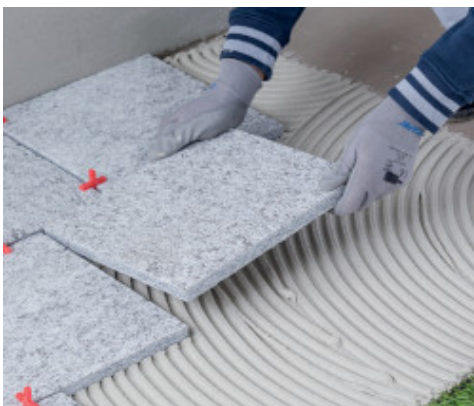
Installation of natural stone in exterior
