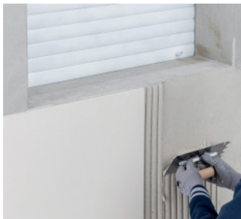
Installation of large-size ceramic tiles
